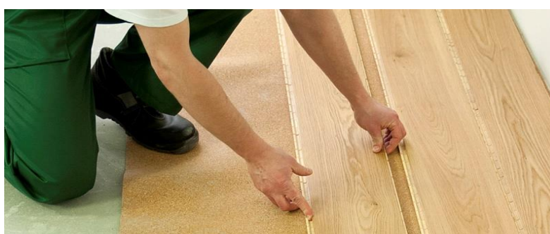
Fig. 3. The view of 3-layer wooden floorboard during installation
